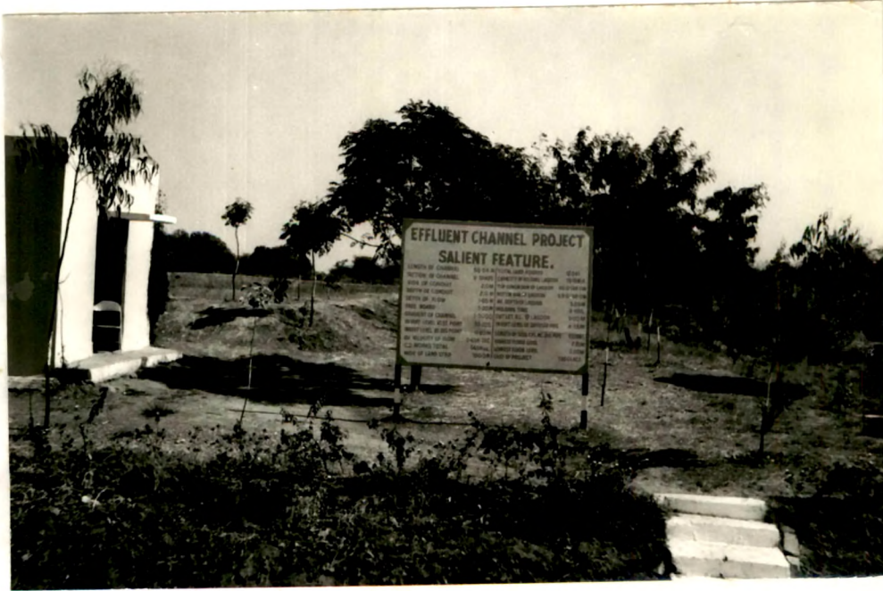
PLATE VI.6 A view of showing the effluent channel project, Loc. near Sarod
