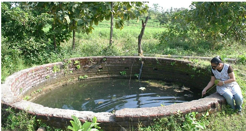
Plate 7. 3b A View of a Lined Open Dug well of Free Flowing Nature developed within Weathered Basaltic Aquifer in a Pediment Zone( Loc. Tadphalia)
