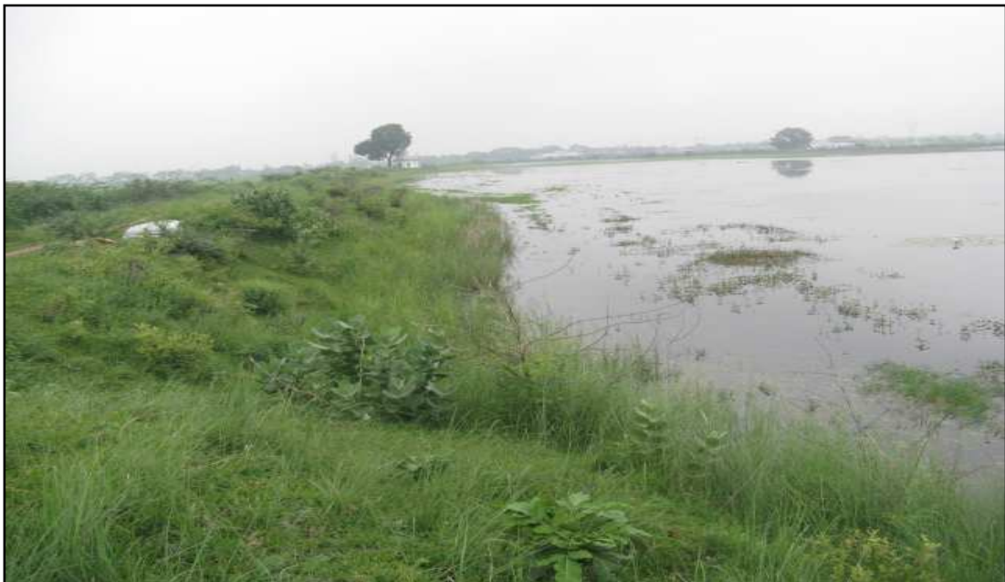
Dense vegetation covering the earthen dam during monsoon
