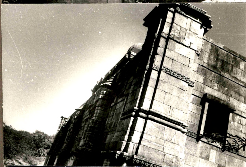
→ Qibla Wall with buttresses
