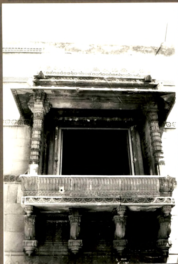
Balcony (Southern end)
