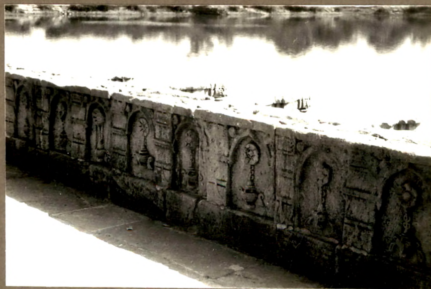
wall over inlet sulice
