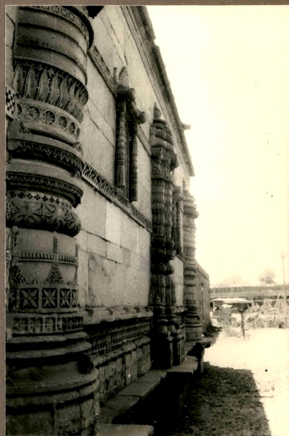
Qibla Wall with buttresses
