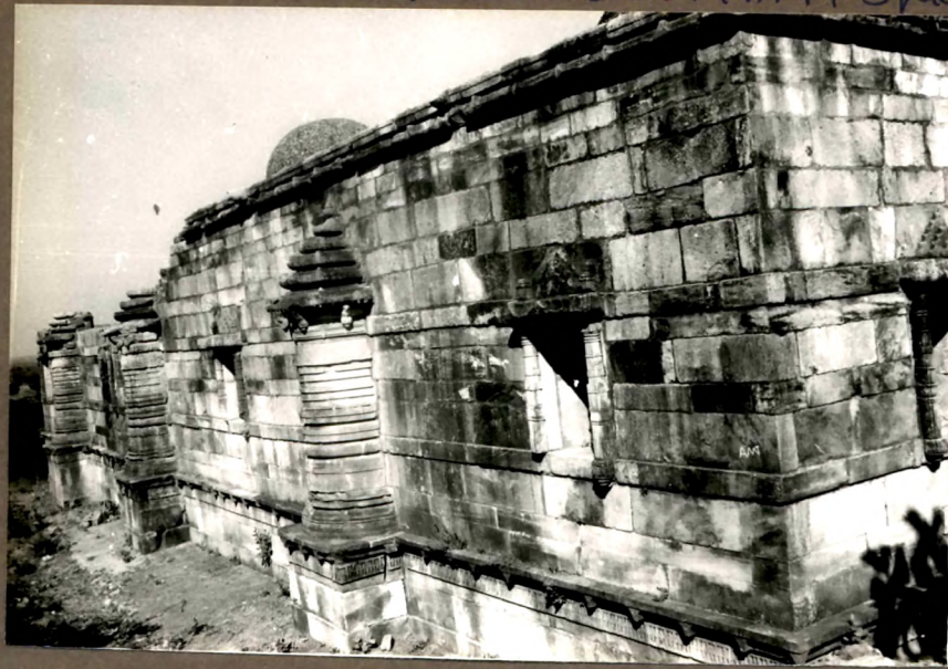
Gibla Wall with buttresses: Bauwamin Mosque
