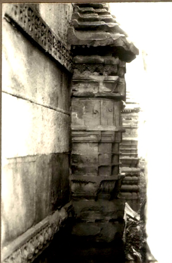
Buttresses on the Qibla wall
