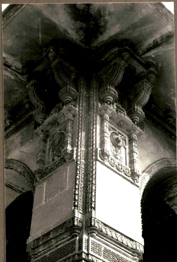
Upper shaft and pillar capital
