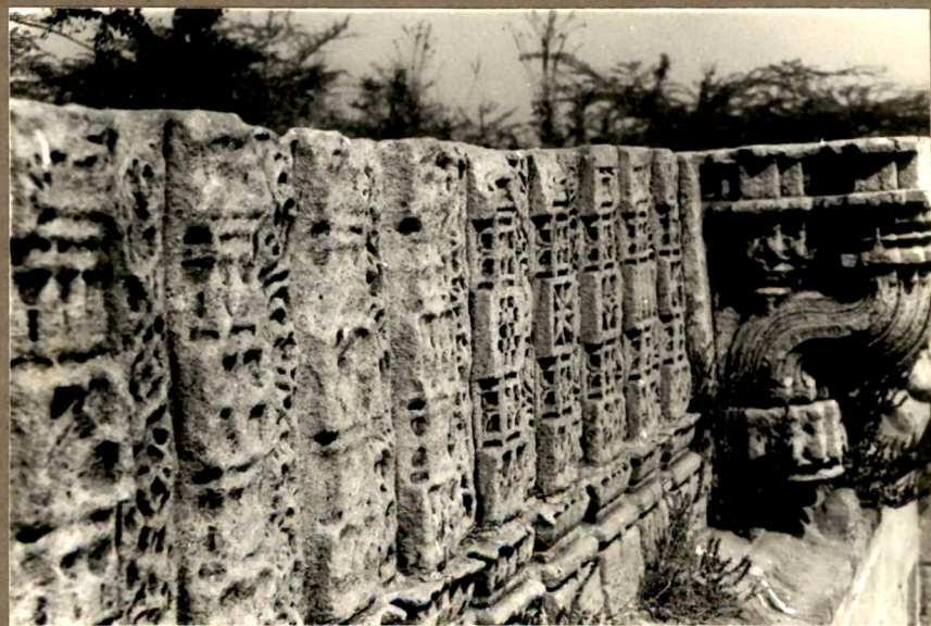
wall & bracket over inlet sulice
