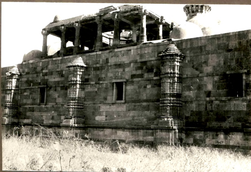
Qibla Wall with battresses : Kewara Mosque
