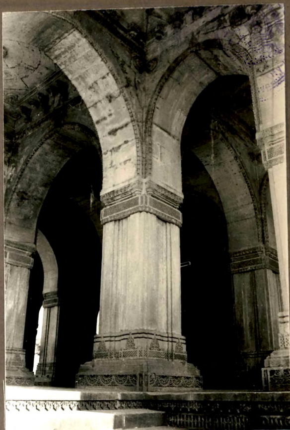
Detail of porch
