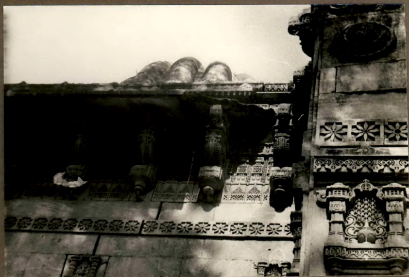
Eaves and brackets
