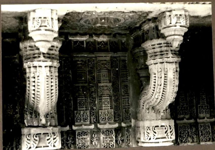
Bracket under balcony.
