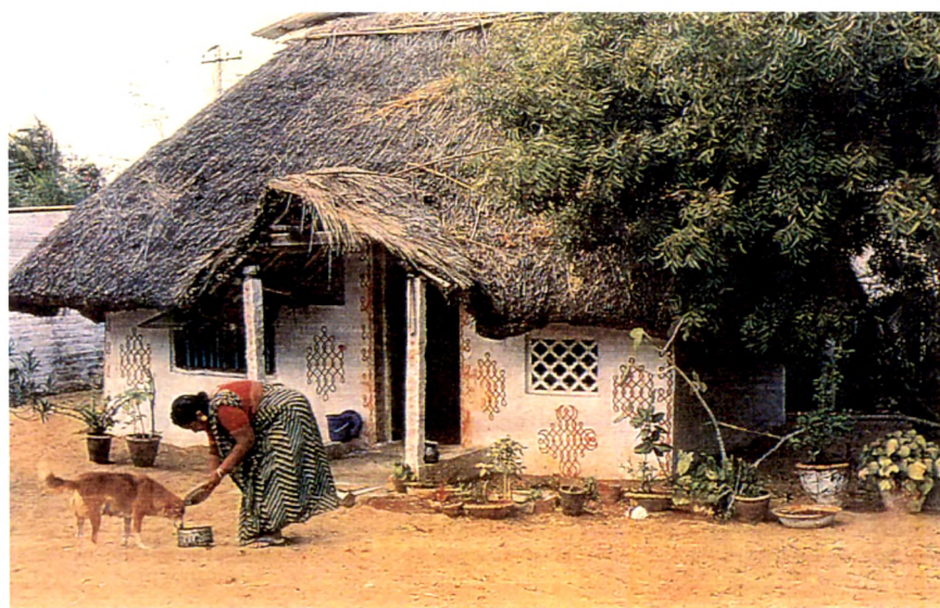
Fig. 41. A house at Cholamandal, with masonry walls and thatched roof
