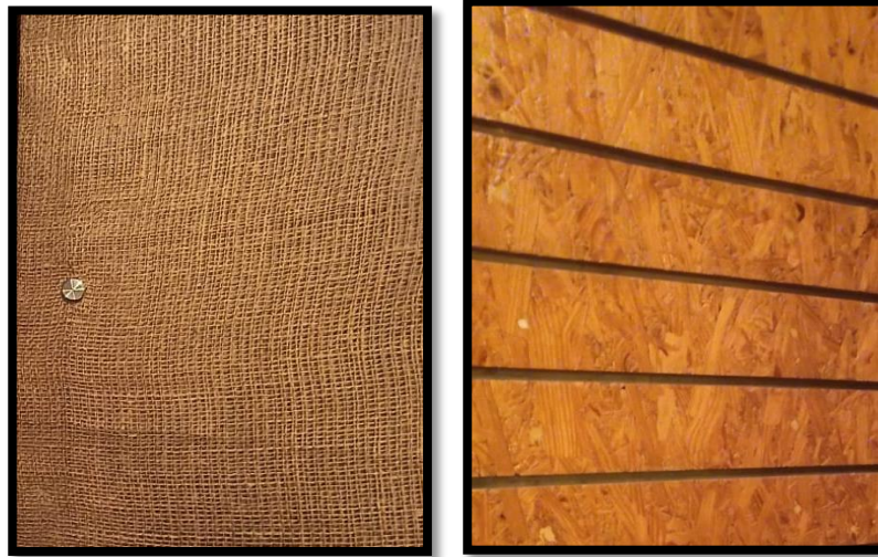
Plate-12 Existing acoustic treatment on the walls of theatre room
