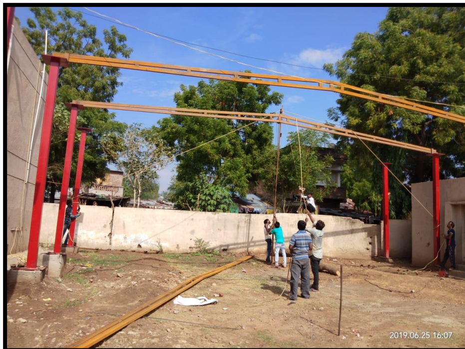
Plate 28: INSTALLATION OF PEB STRUCTURE IN MID-DAY MEAL AREA OF THE SCHOOL
