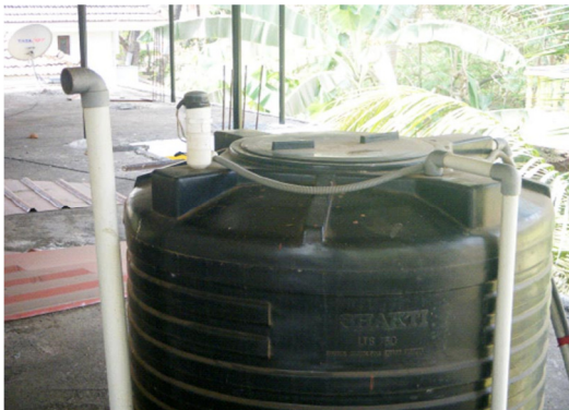
Plate 18: Installed water level controller in water tanks
