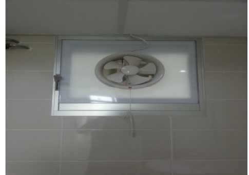
Plate 29: Exhaust fan in bathroom
