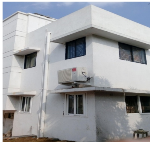
Plate 23: Weather shed windows constructed to reduce afternoon heat entering the house
