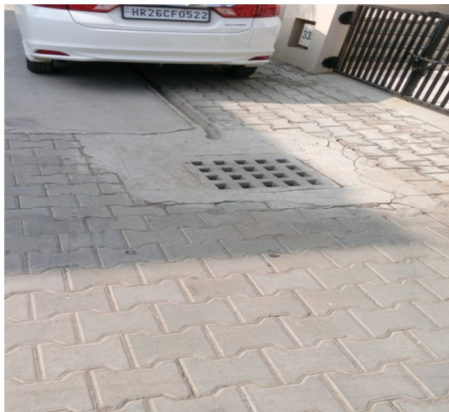
Plate 12: Impermeable Surface directing all run off towards Storm water collection pit
