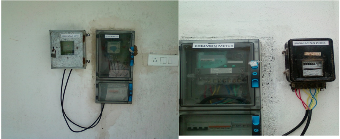
Plate 17: Installed submeters for various water usage
