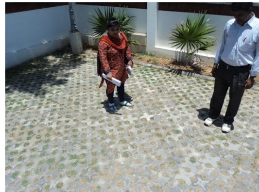
Plate 13: Paved area constructed with permeable paving
