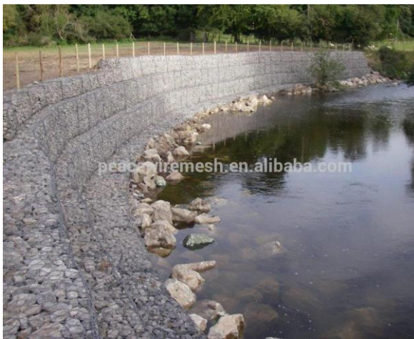
Figure 20: Gabions as retaining wall
