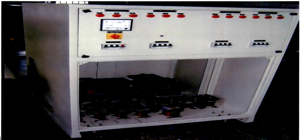
Photo A-II.8: Signal Conditioning Block for input to ADC
