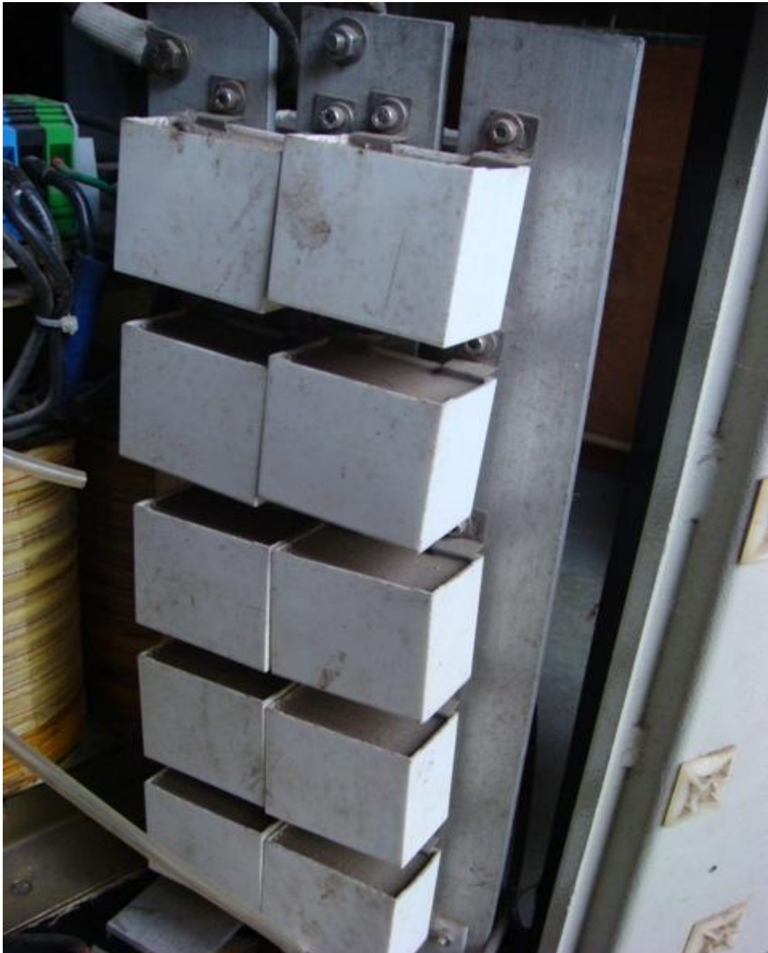
Figure 5-1 Tank Capacitor Bank
