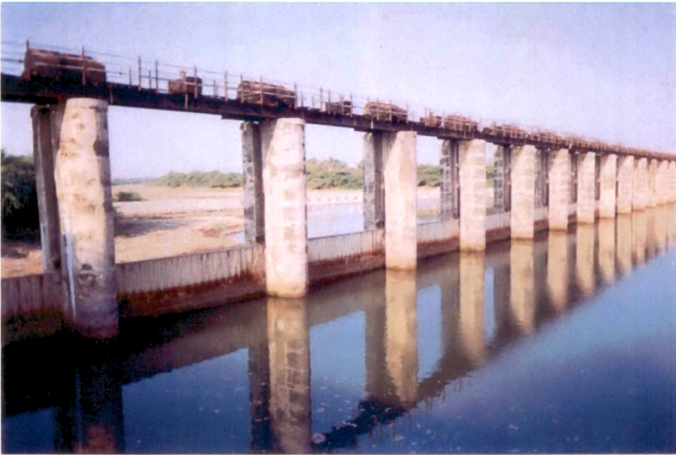
Plate 4.7: View of Mul Dwarka Tidal Regulator Gate from D/S Side
