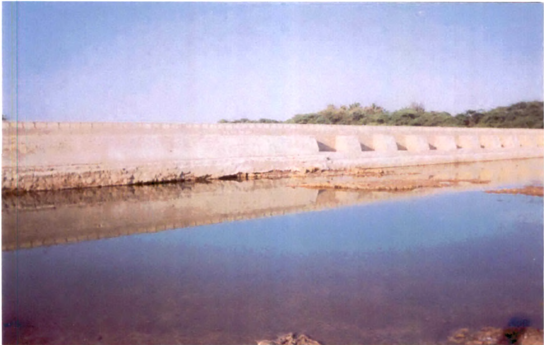
Plate 4.9: Close view of U/S Weir
