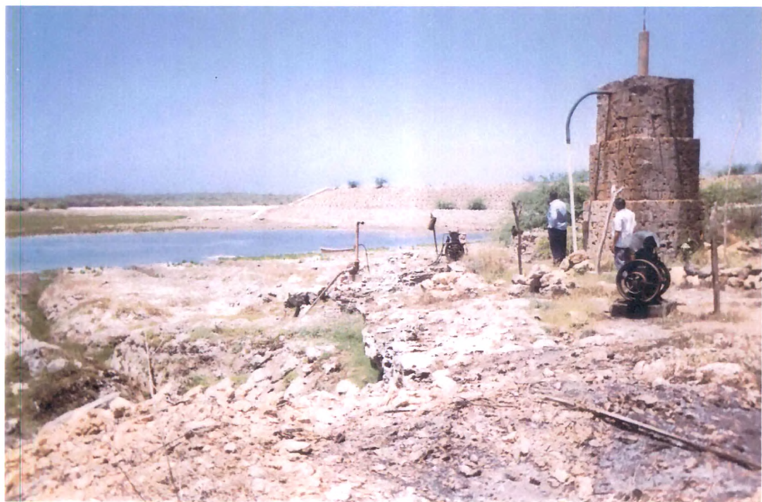
Plate 4.16: View of Shardagram Bandhara from U/S Side (On U/S side Pumping Masonry Tower is visible to supply water directly from reservoir to Farm)
