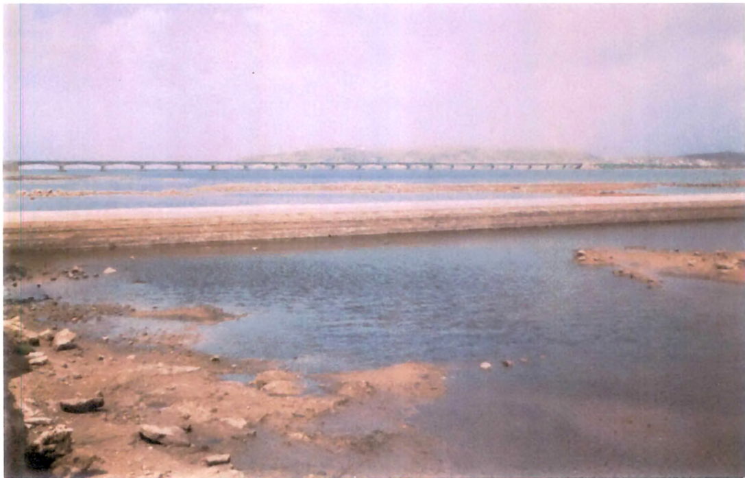
Plate 4.1 : View from D/S side Medha Creek Tidal Regulator
