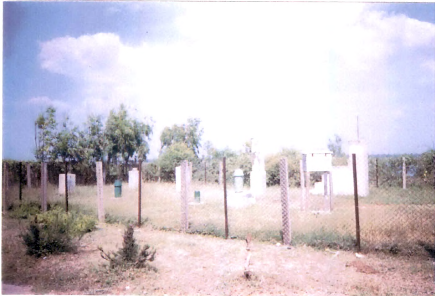
Plate 4.4: View of Meghal Tidal Regulator Hydromet Station
