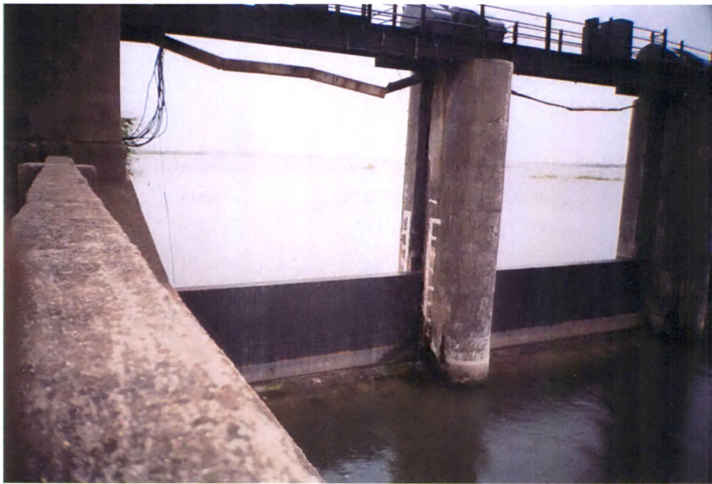
Plate 4.5: View of Meghal Tidal Regulator Gate – U/S & D/S of Reservoir with RL marked on Pier (The colour difference between Fresh Water and Sea water is visualized in the same. U/S side is filled to FRL.)
