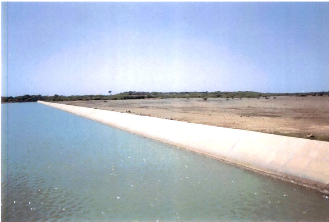
Plate 4.12: View of Barda Bandhara from U/S Side (On U/S side Silting is visible nearly upto height of Bandhara.)
