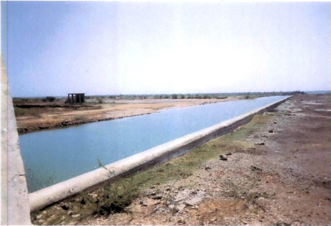
Plate 4.12: View of Barda Bandhara from U/S Side (On U/S side Silting is visible nearly upto height of Bandhara.)
