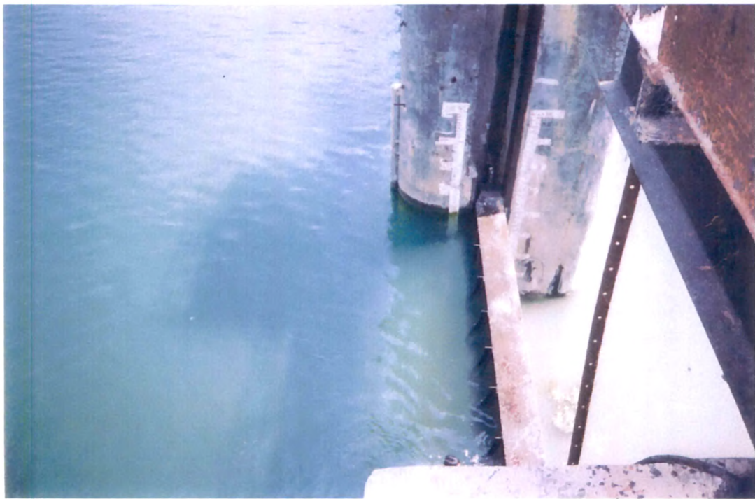
Plate 4.5: View of Meghal Tidal Regulator Gate – U/S & D/S of Reservoir with RL marked on Pier (The colour difference between Fresh Water and Sea water is visualized in the same. U/S side is filled to FRL.)
