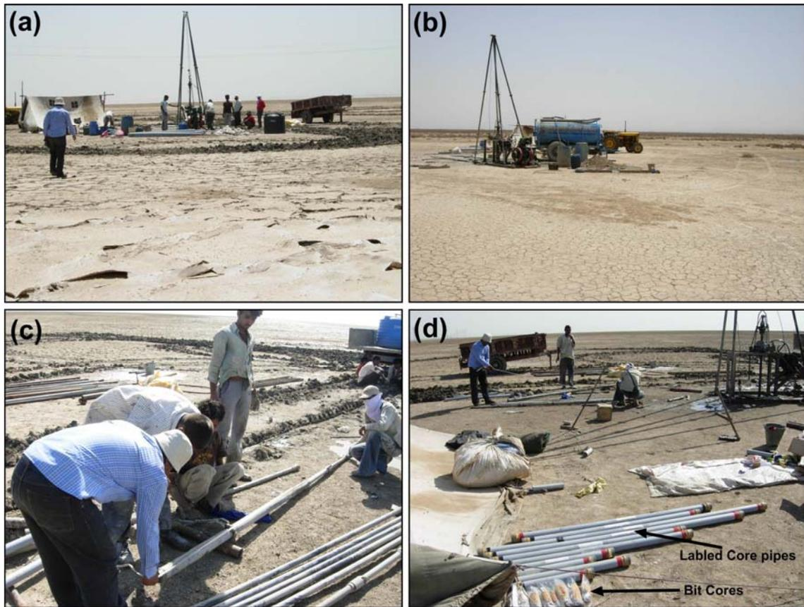
**Figure 2.1** Field photographs showing drilling sites at both the core locations and core pipe measurements during operation. (a) Dhordo Core site, (b) Berada Core site. Please note the foreground at Dhordo drill core site showing the salt encrusted rann surface whereas at Berada drill core site denotes typical banni surface with polygonal cracks on surface. (c) Pipe recovery after drilling and (d) Core recovery measurements, on site logging and packing of individual core pipes.
