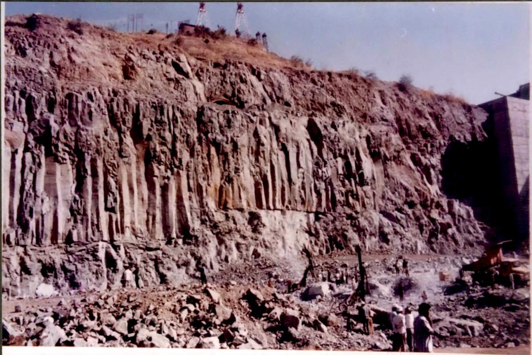
Plate 4: Agglomerate and columnar jointed basalt (basal clinkery zone is absent) in the foundation of right training wall displaced by a fault, Sardar Sarovar (Narmada) Project
