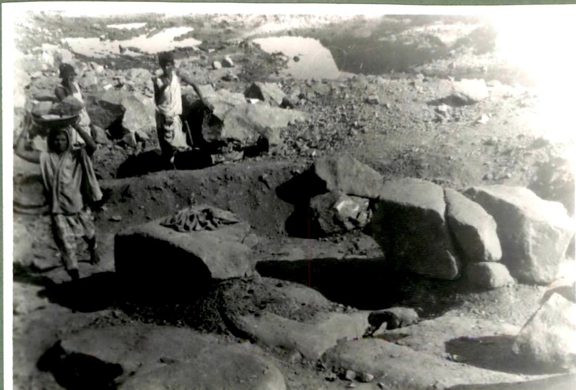
(b) Preparation of in-situ shear test blocks on weathered rock seam
