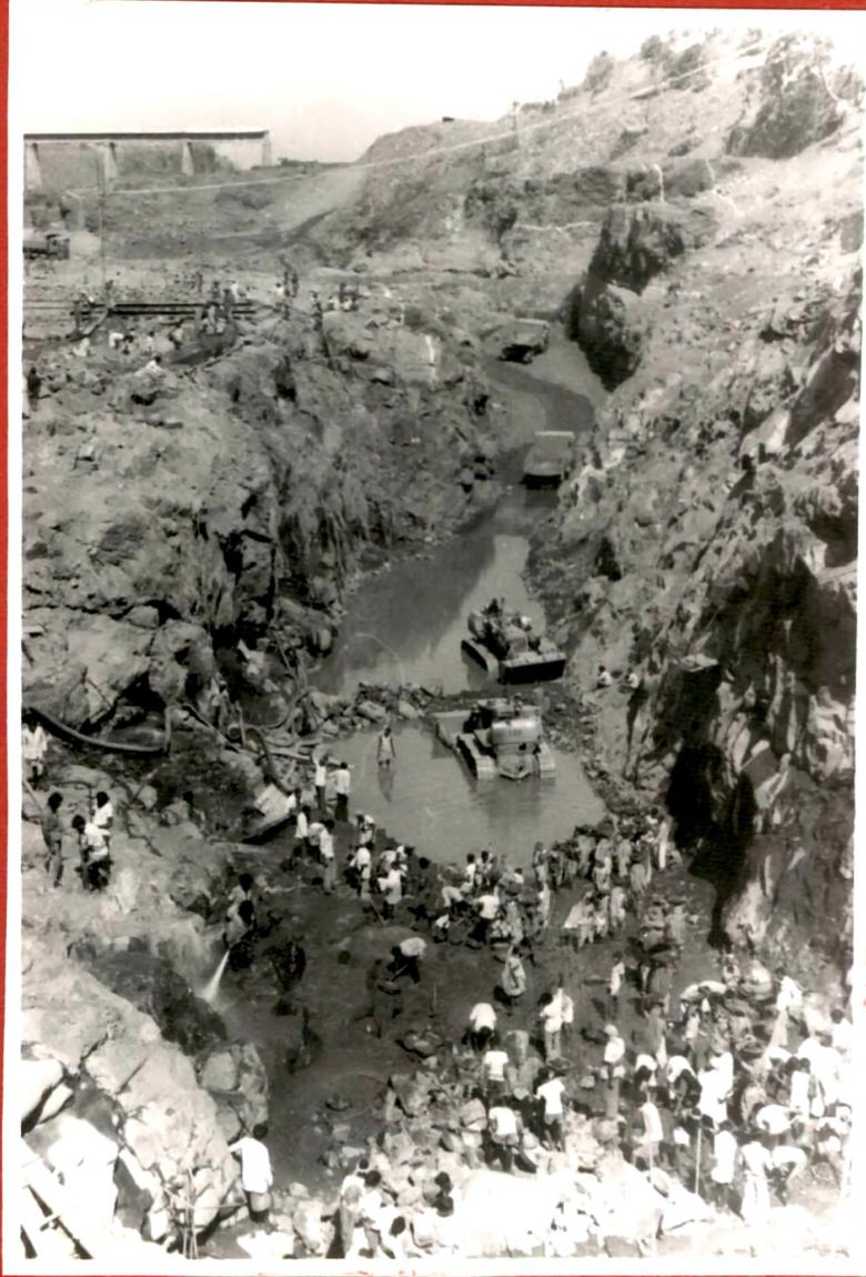
Plate 9: Foundation preparation of the river channel fault exposed at the dam base (view from upstream), Karjan dam
