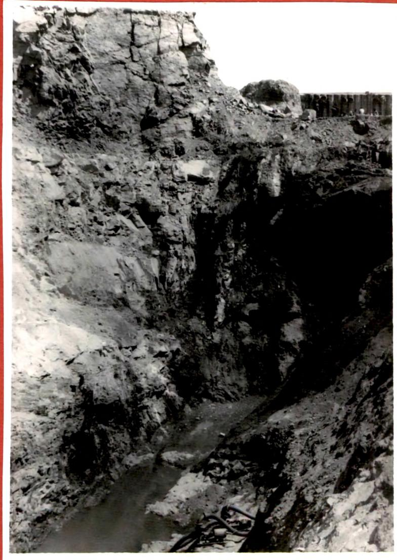
Plate 6: Excavated trench along river channel fault, Sardar Sarovar (Narmada) Project
