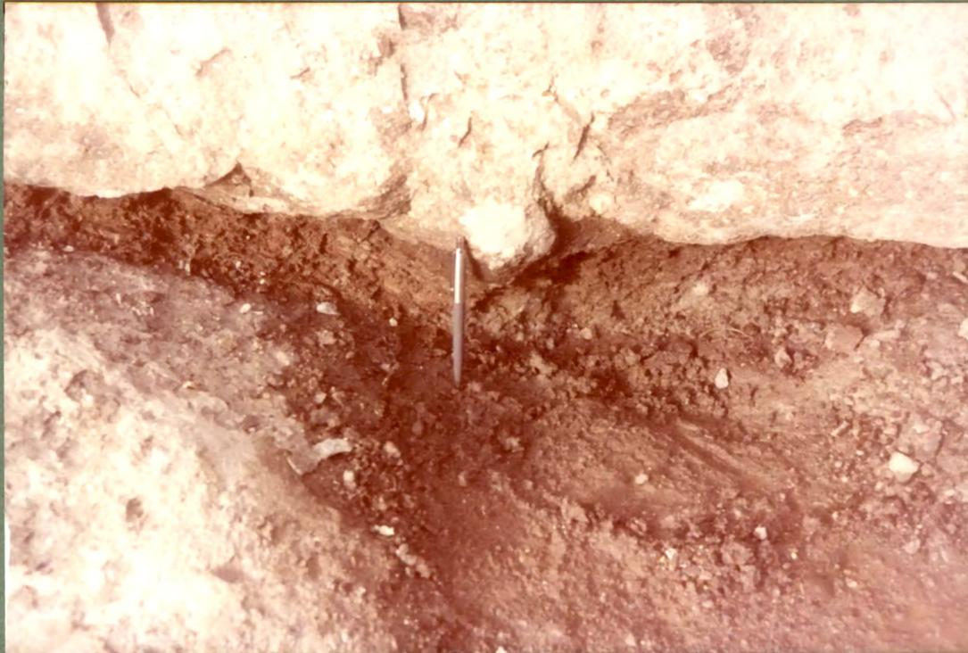
(a) Disposition of weathered rock seam in the foundation of dam block
