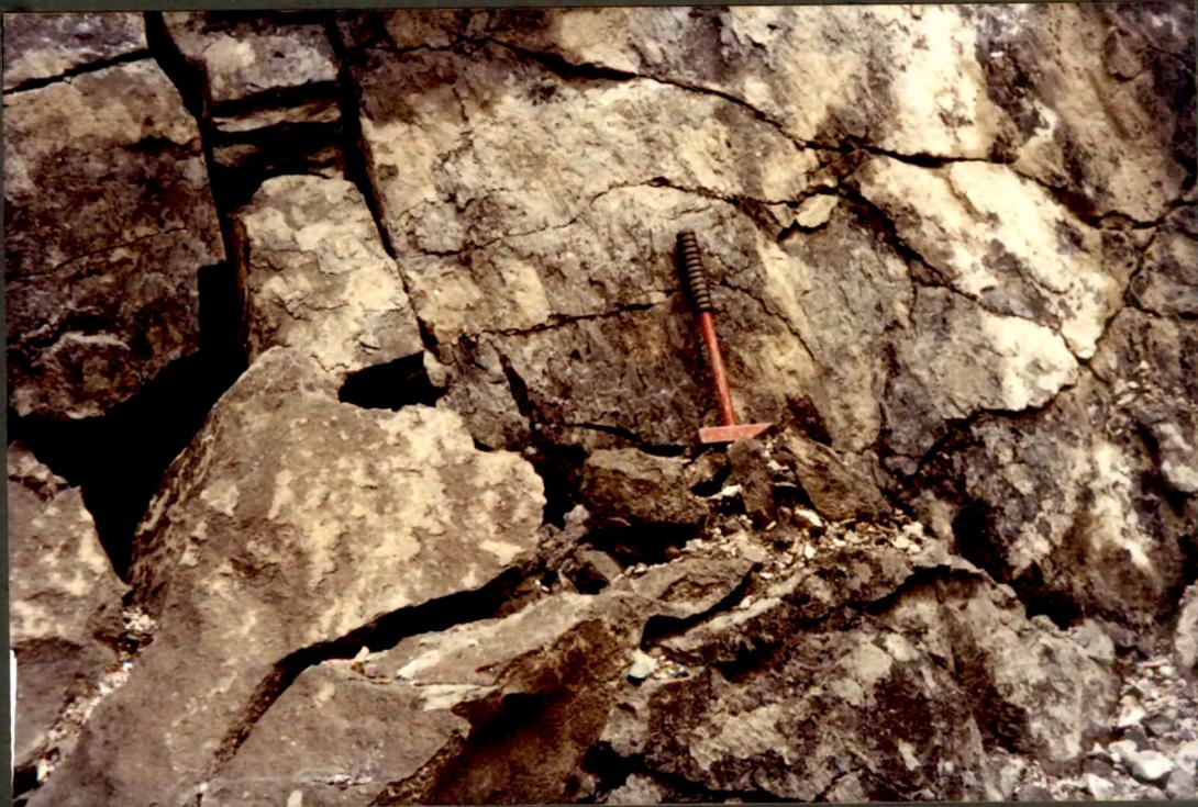
Plate 23: Slaking of dolerite rock at the portal site of Exit Tunnel, Sardar Sarovar (Narmada) Project
