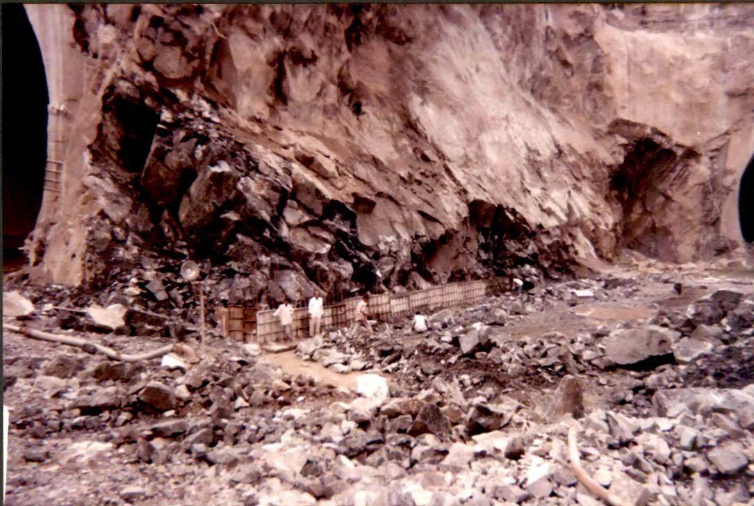
(b) Slaked dolerite sill at the outlet portal site of the tunnel
