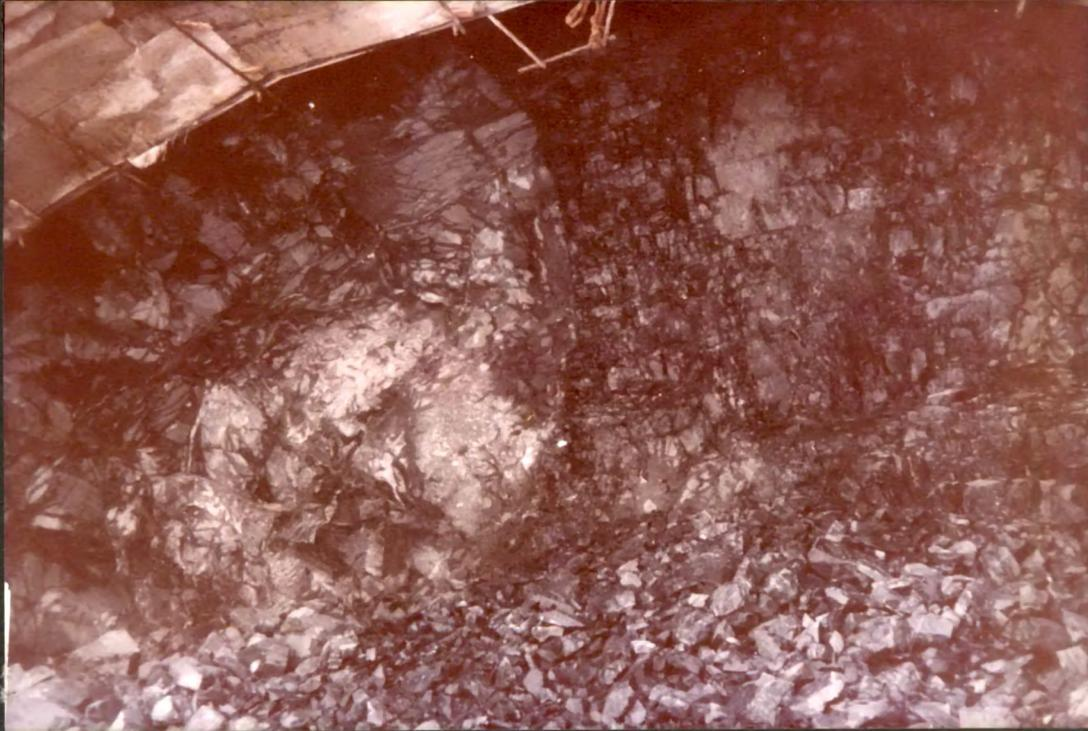
(a) Partly slaked vertical dolerite dyke inside the tunnel
