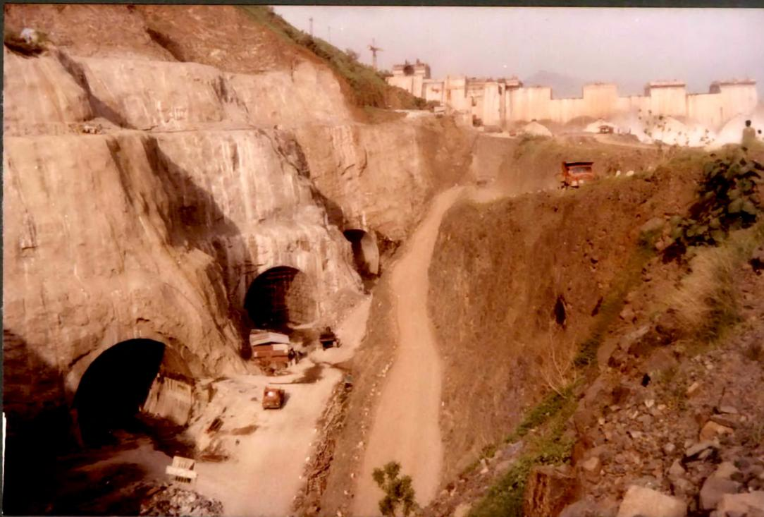
(b) Shotcreted (with wire mesh) outlet portal face of the tunnels
