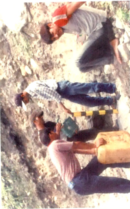
E. Covering with sand from the base of perforation to make a 60cm sand filter column around the perforated pipe section
