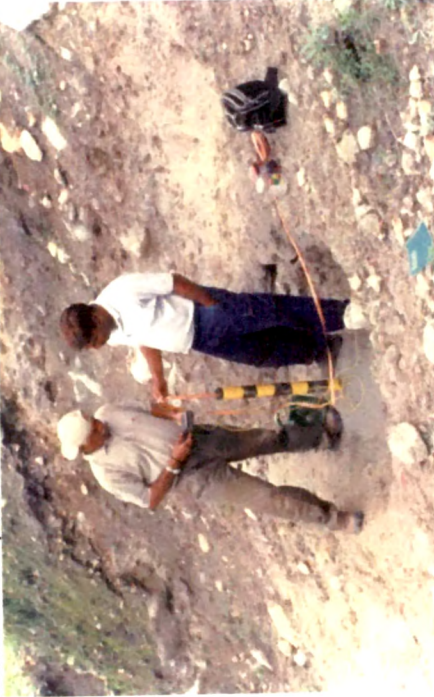
F. Sealing the total 90cm sand filter column with Bentonite Plug to restrict vertical percolation of water into the Piezometer device
