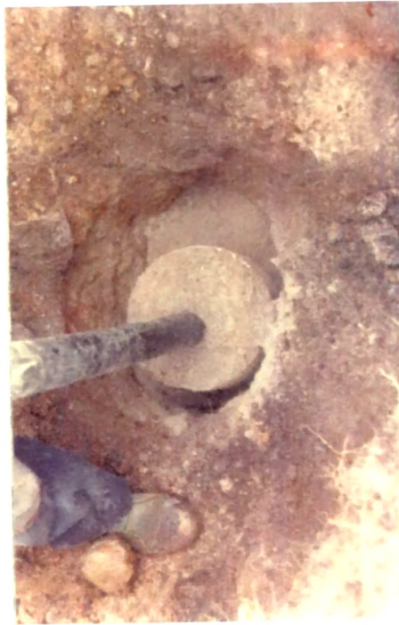
E. Covering with sand from the base of perforation to make a 60cm sand filter column around the perforated pipe section
