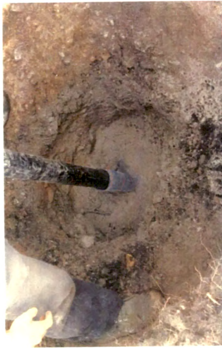
D. Emplacing the perforated pipe wrapped with wire mesh on a base of 30cm sand filter column.
