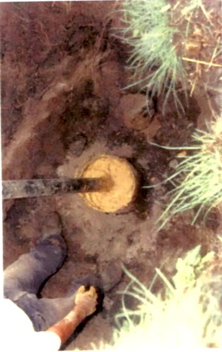
F. Sealing the total 90cm sand filter column with Bentonite Plug to restrict vertical percolation of water into the Piezometer device
