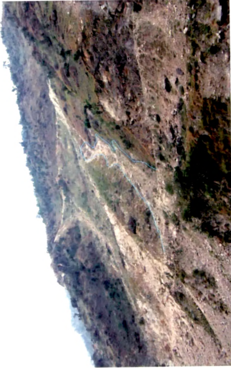
J. Side view of Mangti Landslide from GREF Camp. Blue line shows the periphery of slid mass near the shoulder portion (June 2005)
