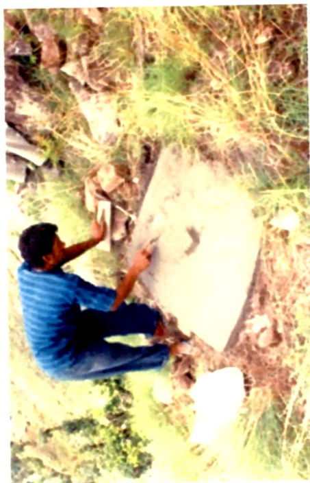
A. Construction of 3'x3' concrete permanent Bench Mark on stable ground
