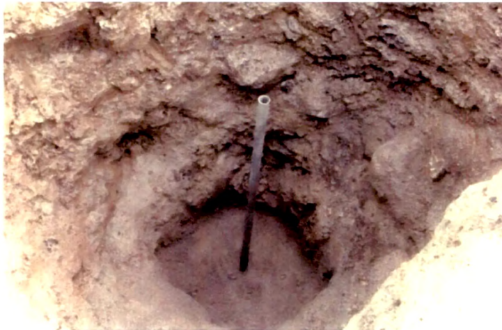
A. Fixing of movement monitoring rod with concrete mix
