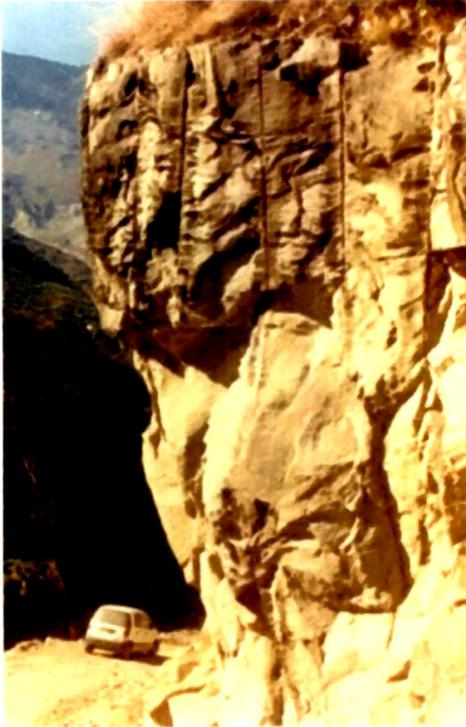
**A.** View of closely spaced blast holes along TJRC
