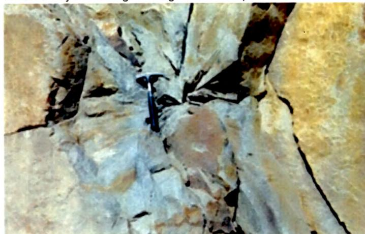
**F.** Field photograph of radiating fractures created in Biotite Gneiss rock in shoulder region of Mangti Landslide on account of uncontrolled blasting carried out during road construction stage
