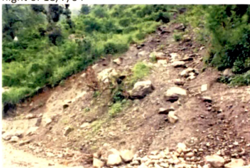
26b. View of a stream flowing through the slide is charging this debris slide and more slope material is seen flowing down and the crown is seen expanding; 22/7/04
