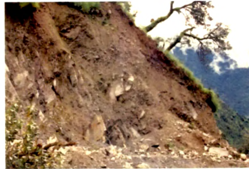
21a. View of discontinuity controlled wedge slide on upper level of road below Galagad village; slide occurred on 22/7/04
