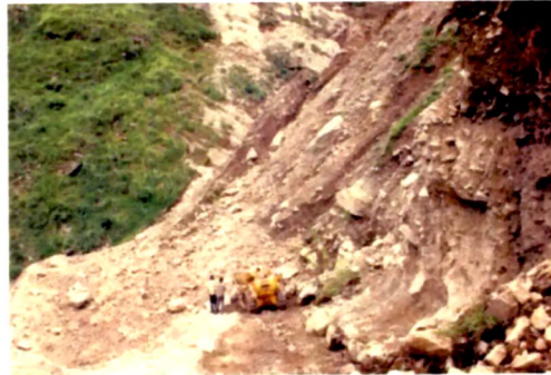
20c. View of dozer clearing the slid material along this newly constructed segment of road
