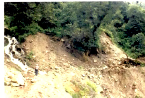
24. View of severely affected newly constructed road stretch below Galagad village with profuse shallow soil slip debris slides; 18/7/04
