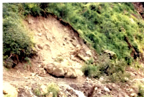
23. View of shallow circular soil slip debris slides blocking the newly constructed road stretch below Galagad village after cloud burst of 18/7/04
