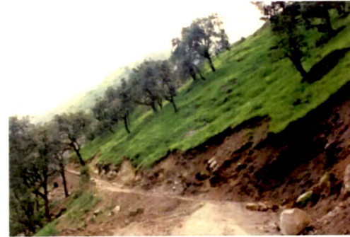
22. Field view of unstable slope showing creep movement; all the trees are seen inclined on the upper level road before Galagad village.
