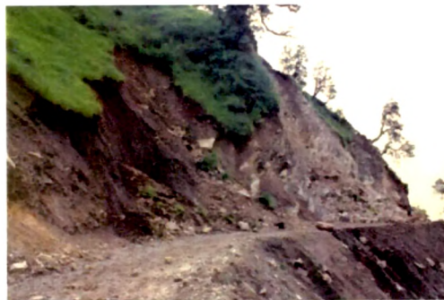
21b. View of laterally expanding shallow soil slips and the expanding wedge slide due to lateral support removal by road construction;dt-18/8/04
