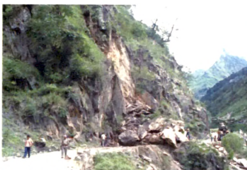
15. View of toppling failure occurred near GREF camp; dt- 17/8/04
