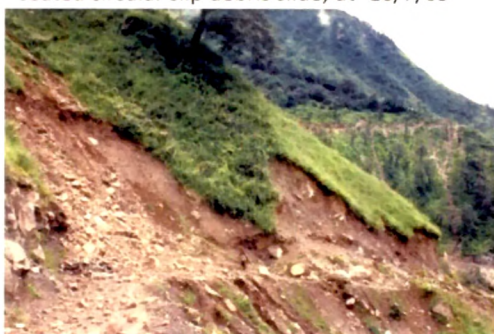
28. View of multiple shallow slip debris slides completely destroying the newly excavated road below Galagad village; dt-18/7/04
