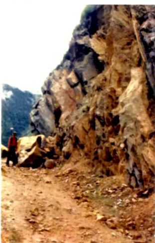
15. View of toppling failure occurred near GREF camp; dt- 17/8/04
