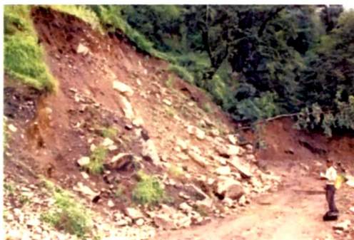
25. View of shallow slip debris slide on the road stretch below Galagad village occurred in the night of 18/7/04
