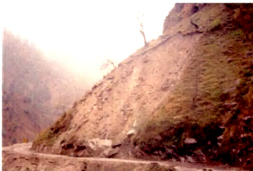
2. View of shallow circular slip debris slide
