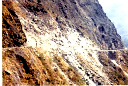
8. View of debris slide in biotite gneiss of CCB at stretch-12 of scanline survey.
