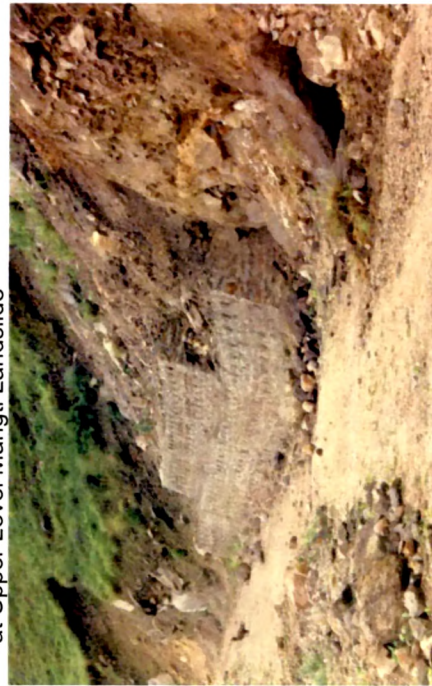
D. View of 4m high constructed Masonry Retaining wall at Upper Level Mangti Landslide
