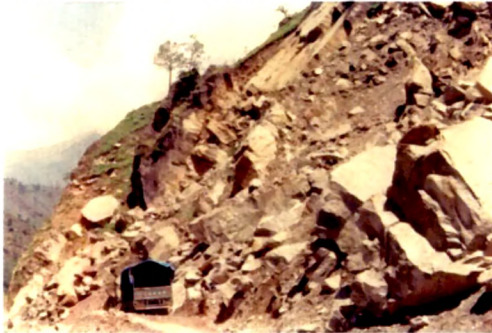
4c. View of the same left flank in June 2004. Surficial material have washed off and huge size rock blocks are seen in critical stage of sliding
