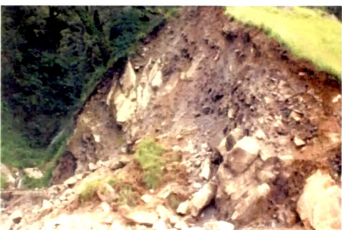
27. View of wedge failure seen completely damaging the road; dt-18/7/04
