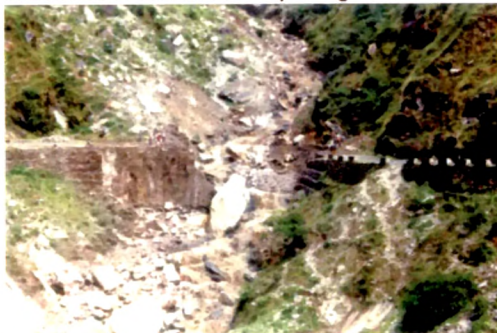
9. View of 30m formation washout occurred due to cloud burst above Pangla village; dt-18/7/2004
