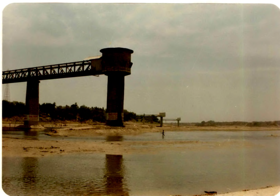
PLATE 26 : VIEW OF ONE OF THE FRENCH-WELL DUG IN THE MAHI-RIVER BED AT FAJALPUR FOR THE SUPPLY OF WATER TO BARODA CITY AND INDUSTRIES. THE MEAGRE WATER QUANTITY IN THE RIVER IS CONSPICUOUS.
