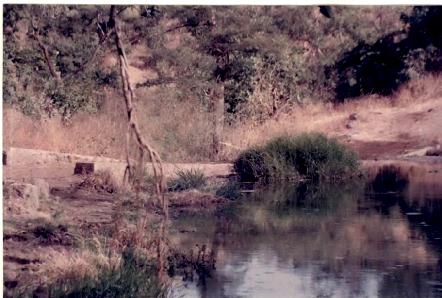
Plate 36 - Blockage of stream by causeway.
