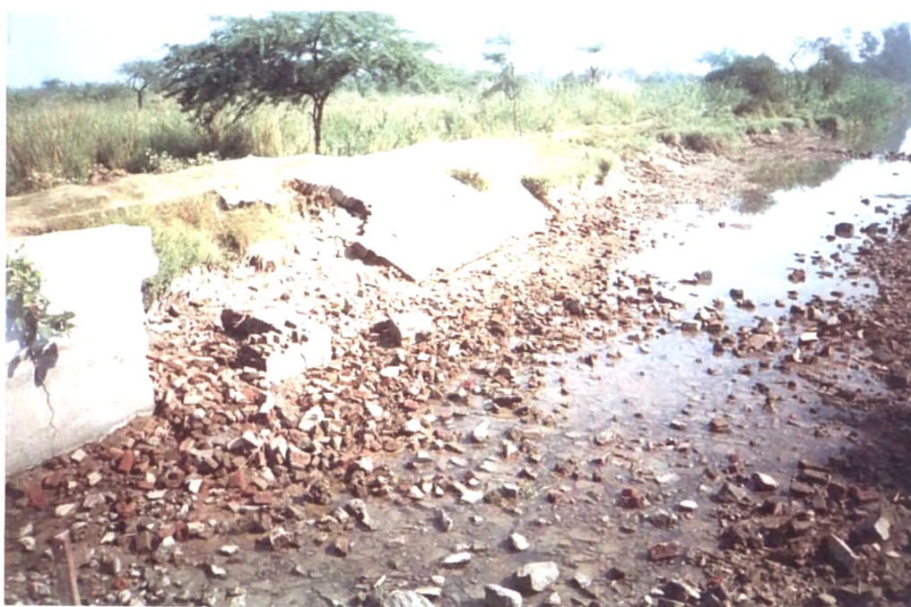
Plate 9 Damaged Embankment Structure of Canal of Chalthan Branch Canal (Loc. Near Mota village).
