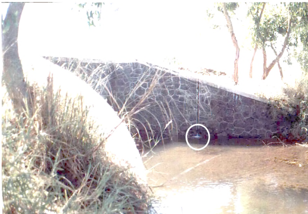
Plate 7 Seepage Through Canal Structure Causing Water Ponding.
