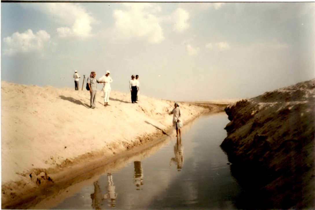
Plate 6.5 a Thick sands in Banas bed as seen in foundation excavation for underground checkdam near Badarpura village
