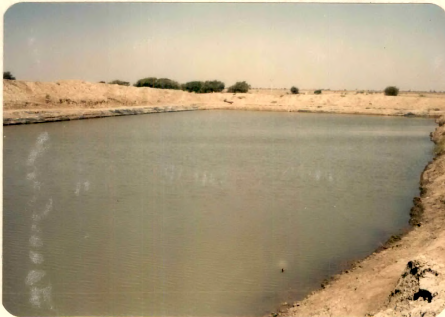
Plate VII.6. An artificial polypropylene lined pond for sweet water storage at Rahtalav.
