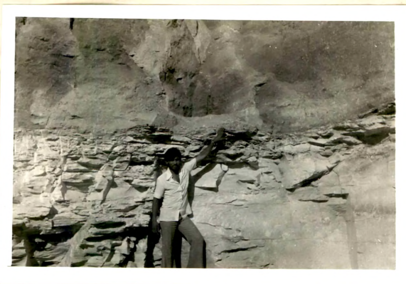
Joints in fireclay below compact finegrained sandstone.
