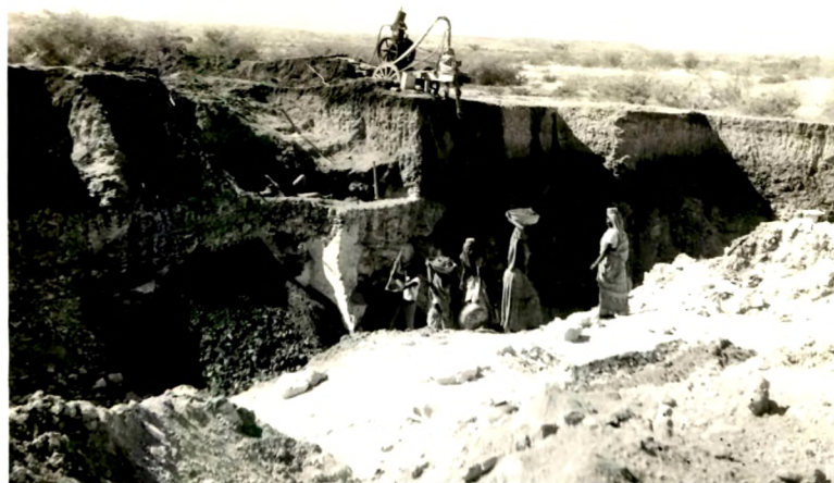
Pumping of water from the mine pit to keep it working.
