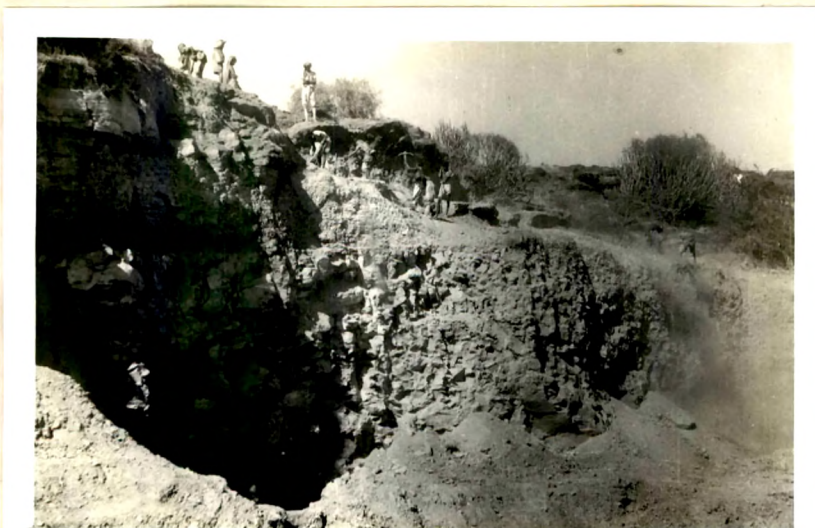
Semi-flint to flint clay showing greatest thickness (9.6m).
