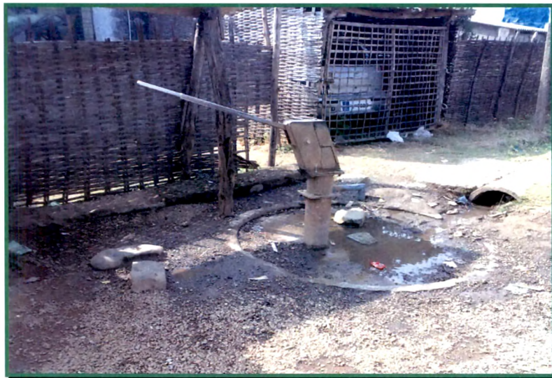
Plate 4.6 – The improperly maintained bore well in the school
