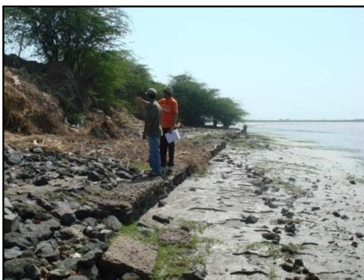
Damaged sea wall at Kaladara (Vagra)
