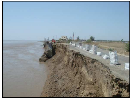
Erosion of road at Kaladara (Vagra)
