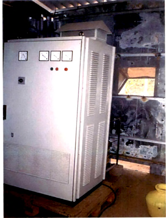
Fig 3.21 (c) STATCON installation in site at Nagercoil (TN), India on 250kW windmill
