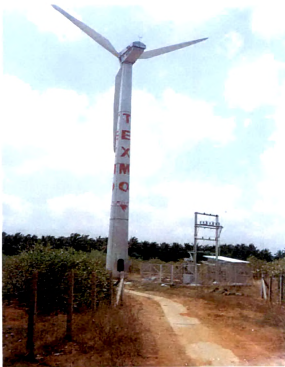
Fig 3.21 (c) STATCON installation in site at Nagercoil (TN), India on 250kW windmill
