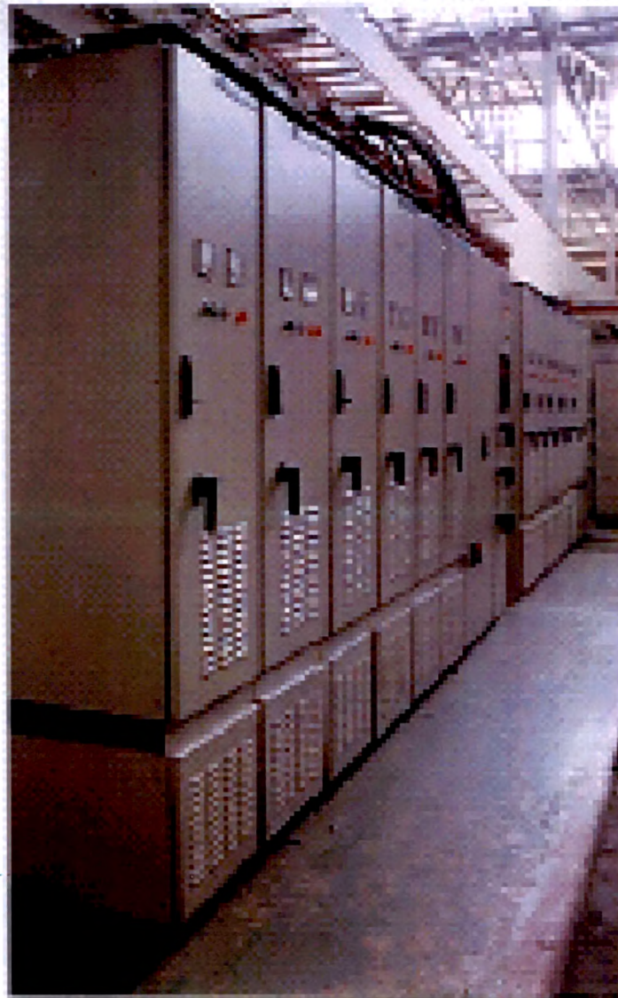
Fig 3.31 (c) STATCON installation in automotive industry
