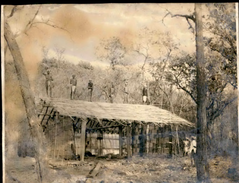
Thatching a cattle-byre under construction.
