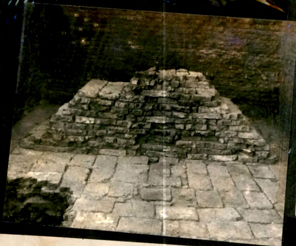
22. Stupa : Section of stepped structure in core of the Stupa.
