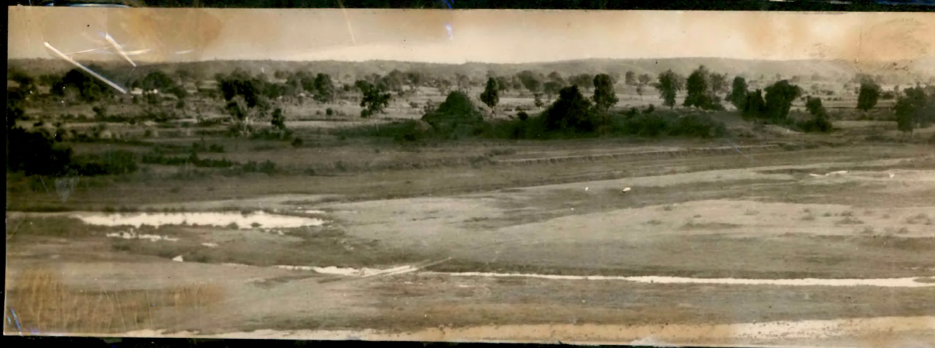
3. The site from north-west.
