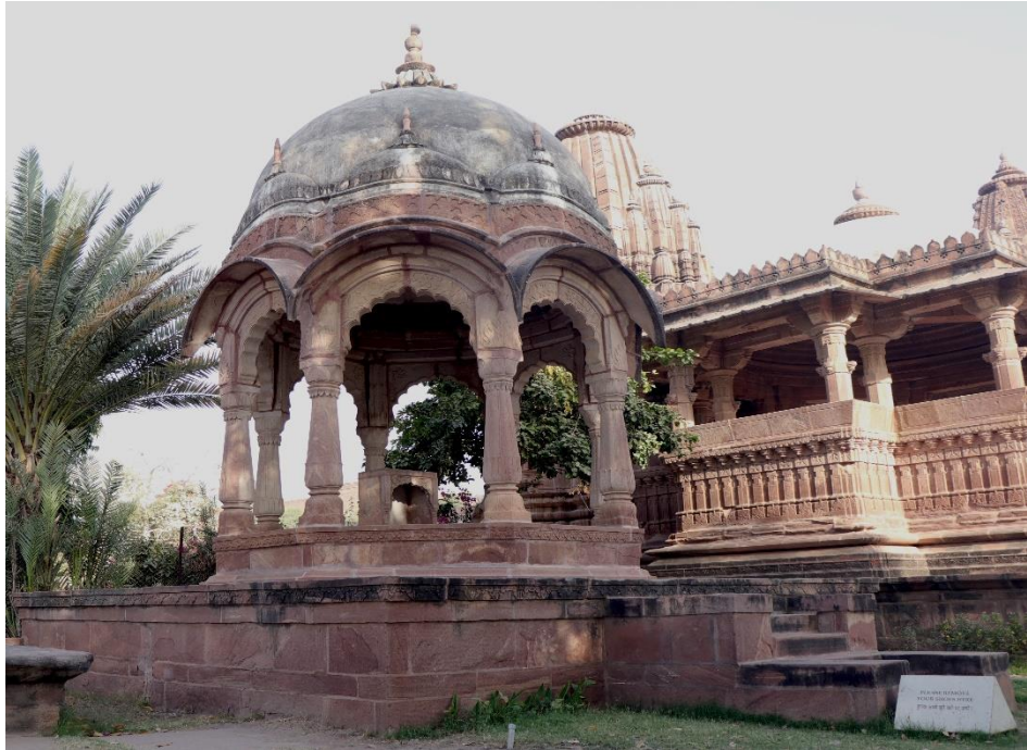
Plate 2.57 Angular view Chatarī of Bāijī Lāl Abhē Kamwar , Maṁdor , Jodhpur , Rājasthān .
