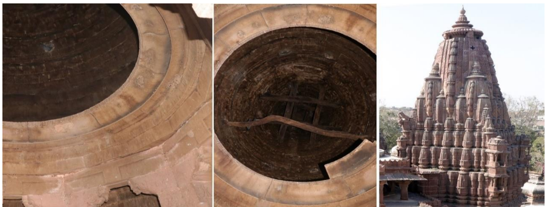
Plate 4.14 (Left) Interior wall of Śikhara resting on the ring and coloumns, (Center) Interior view of Śikhara , (Right) Exterior view of Śikhara .
