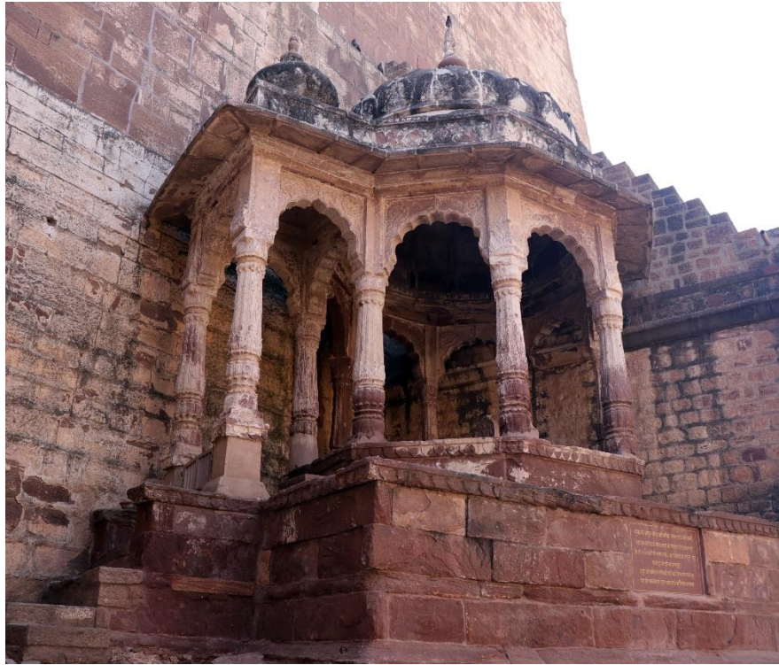
Plate 2.68 Back side view, Chatarī of Kiratsimha , Mēhrāngadhā , Jodhpur , Rājasthān .
