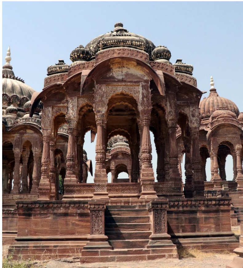
Plate 2.33 Façade, Chatarī of Rānī Vadan Kamwar Cāvaḍī, Paṃcakumḍā , Jodhpur, Rājasthān.
