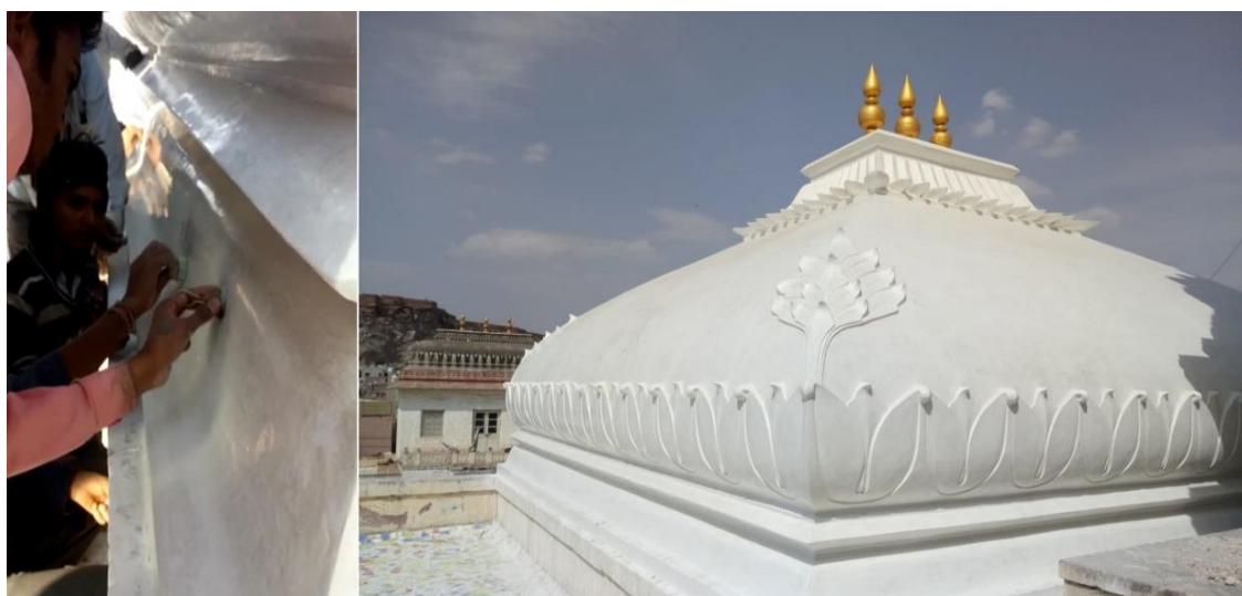
Plate 4.19 (Left) Ghuṭāi process on the lime based Kauḍī plaster, (Right) Final output of Chala dome with Kauḍī plaster
